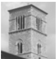
16. Terni Steeple, San Francesco Church
