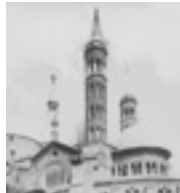
8. Padova Steeple, Basilica of Sant' Antonio
